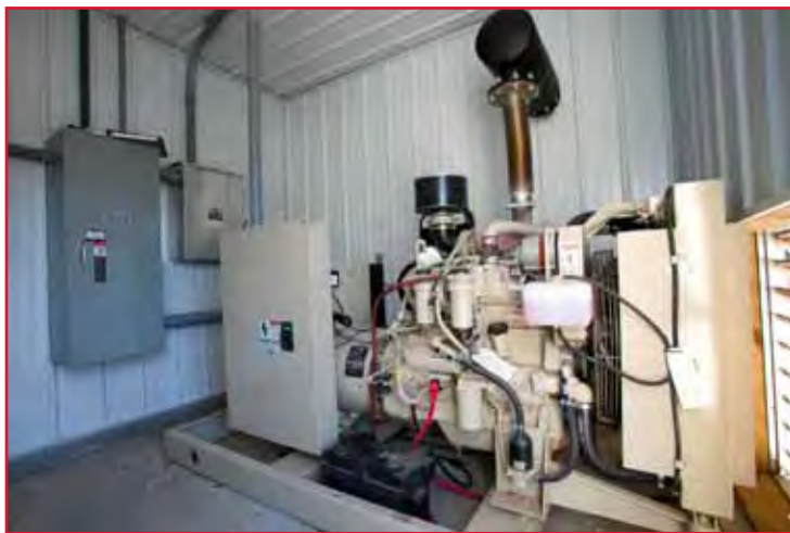
Figure 99: Example of a back-up generator.
