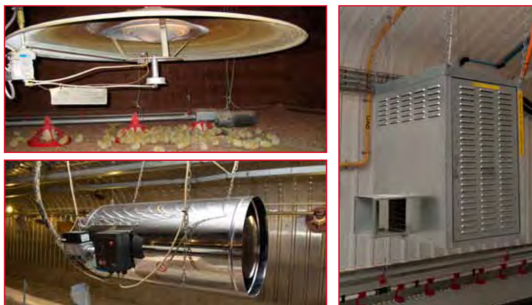
Figure 100: Examples of different house heating systems ( top left - canopy brooder, bottom left - whole-house heating, right - space heater).
